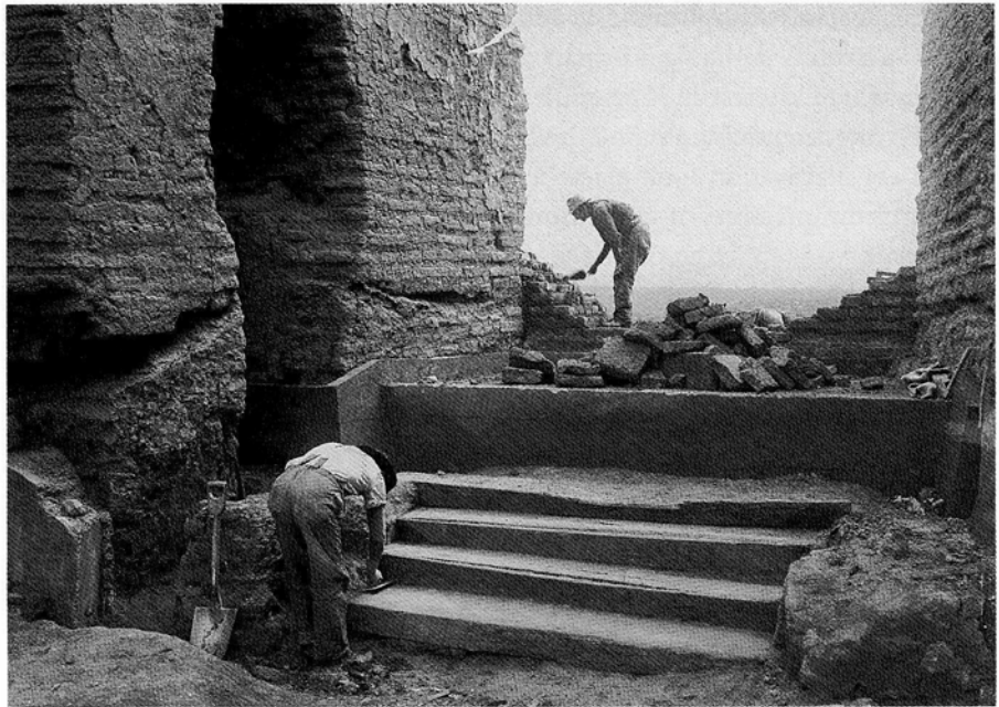
Altar steps of the mission ruin at Pecos during stabilization, 1915.
